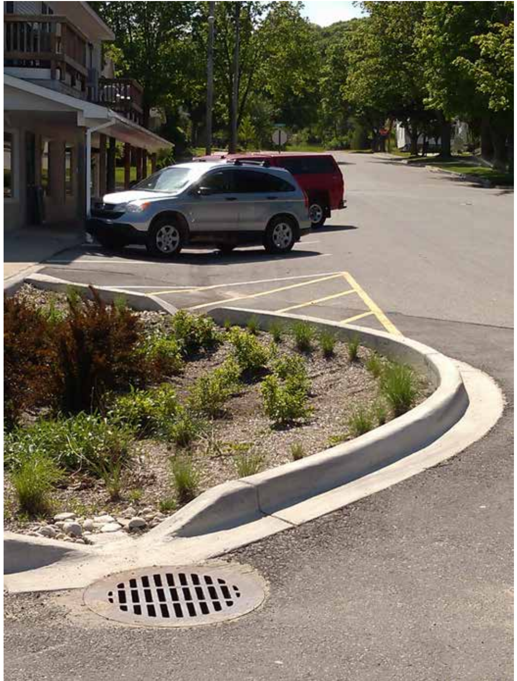
Planning for stormwater management can include controlling the amount, quality, and timing of runoff to prevent its damaging effects on natural resources. Curb cut-outs allow stormwater to flow into this garden and soak into the ground. This helps clean the water before soaking into the ground. The storm sewer allows for overflows to prevent flooding. Photo: DEQ
