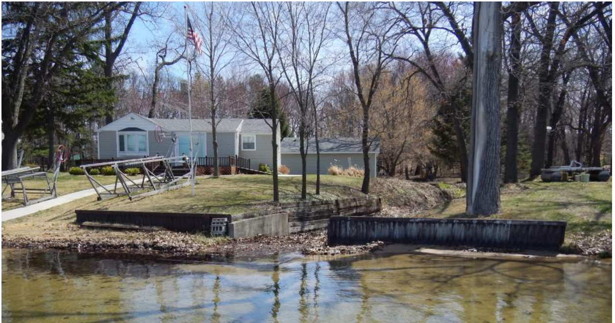
Figure 19. Gravel Lake level control structure and adjacent embankment sheet piling.
